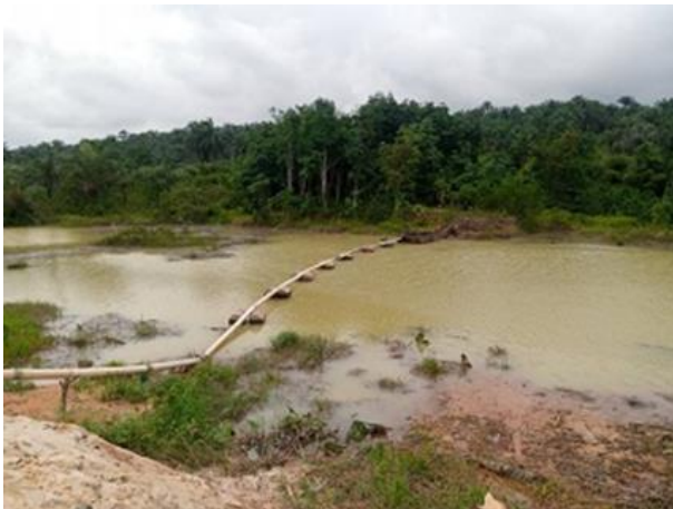
Plate 1: Dredging Machine at work in Anyang Nsit River
